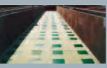
Figure 1: Foundation tank before installing the vibration isolation pads
