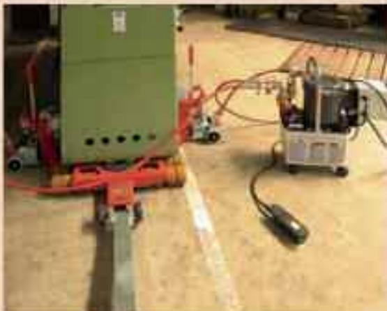
Electric pump JPE 30-NVR with 2 jacks in operation
